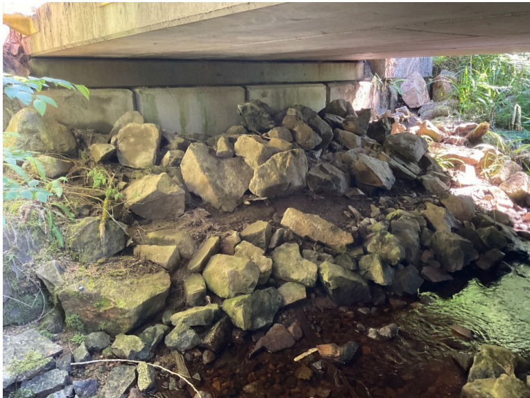
Right Bank Abutment when facing downstream
