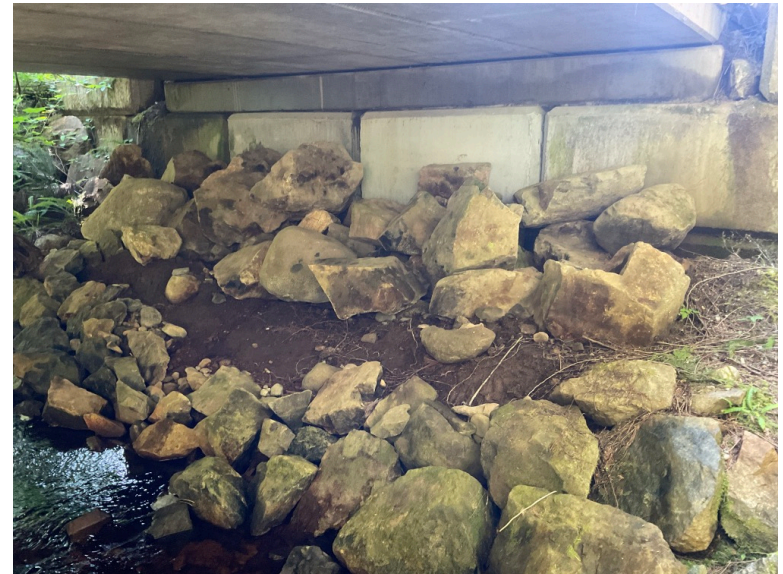
Left Bank Abutment when facing downstream
